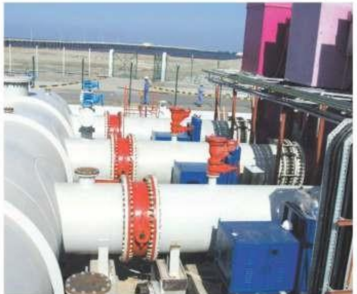
2200 mm Butterfly Valve for Sohar Sea Water Intake Pipeline Project, Oman
