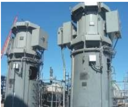
Bechtel- Texas, USA Circulating Water Pumps for 565 MW-Sandow-5 electric station
