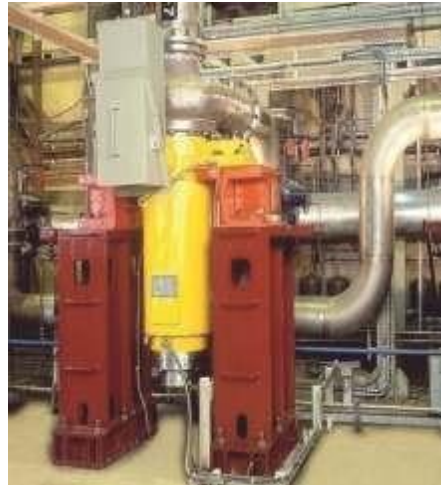
India's first Canned Motor Pump
