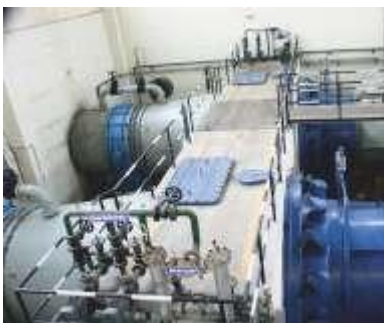
Kerala State Electricity Board, Thiruvananthapuram Ranni Perunad (2 x 2000 kW) HEP Horizontal Kaplan S type
