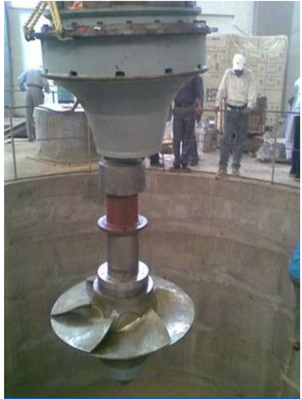
Erection of Vertical Kaplan Runner
