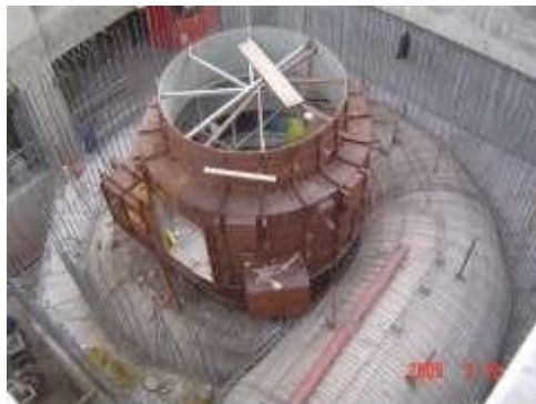
Erection of Casing & Pit Liner
