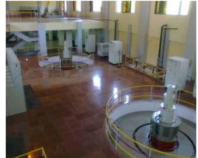
Konal HEP, 2 X 5.5 MW Vertical Kaplan Turbine
