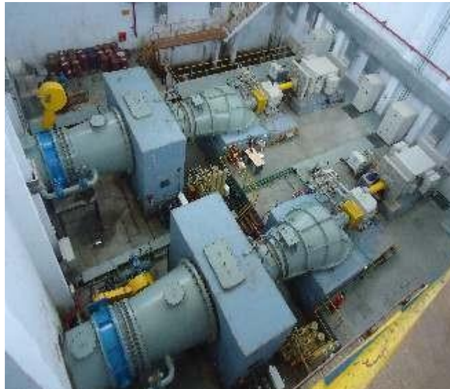
Darna HEP 2 X 2.45 MW, Horizontal 's' Type Tubular Kaplan Turbine
