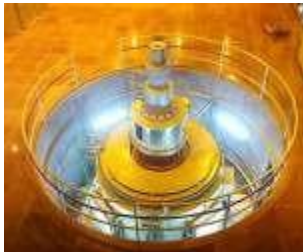
Erection of Vertical Generator
