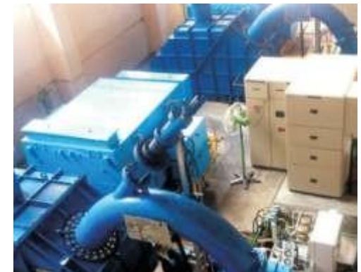
Horizontal Pelton Turbine
