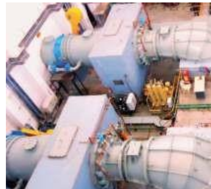
Horizontal Kaplan Turbine
