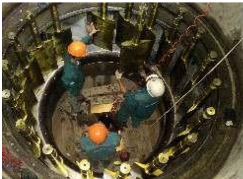
Guide Vane Assembly at Site
