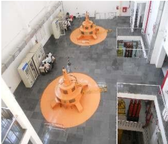
Ankhe Kanak HEP, Vietnam 2 X 6.5 MW, Vertical Kaplan Turbine
