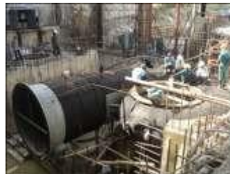
Erection of Spiral Casing
