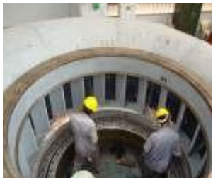
Erection of Stay Ring
