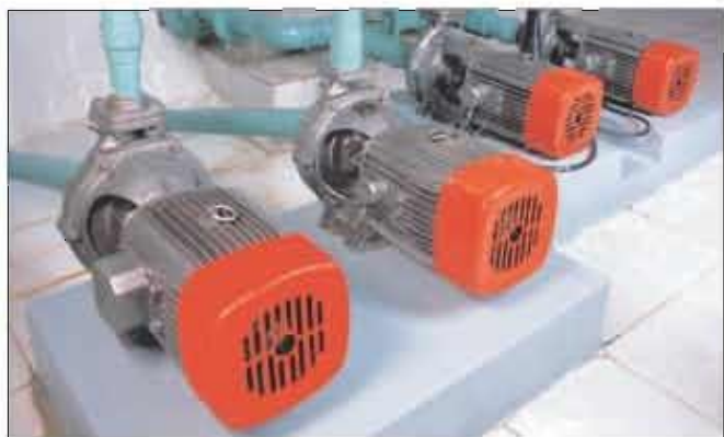
Monobloc Pump in use for water supply at a site in india
