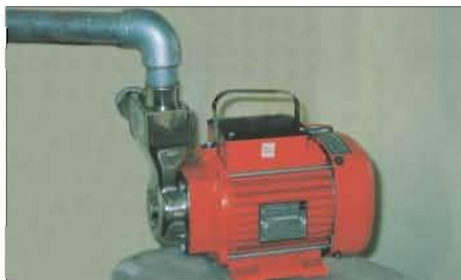
A Monobloc Pump in Stainless steel construction in use for domestic water supply.
