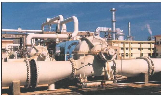
Horizontal Splitcase Pump installed at a Chemical plant in Kochi, India.
