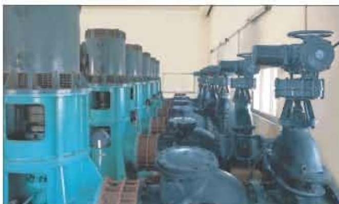
Sluice and Reflux Valves installed at a Metro Municipal Corporation in India.
