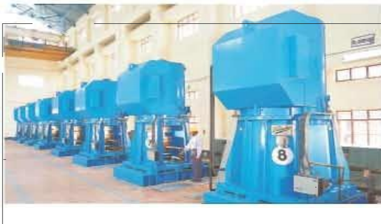
Vertical Turbine Pumps installed at Takari II Stage Irrigation Project, Maharashtra, India
