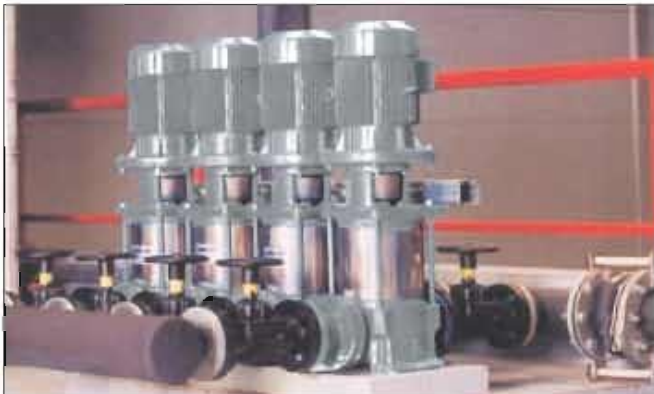
Vertical Multistage pressed stainless steel Inline Pumps installed at a site.
