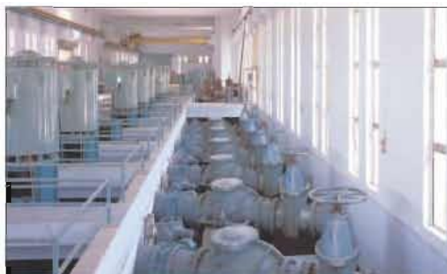
Valves with Pumps installed at Maharashtra Industrial Development Corporation Water Supply Project, Mumbai, India
