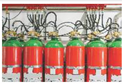
INERT GAS SUPPRESSION SYSTEM
