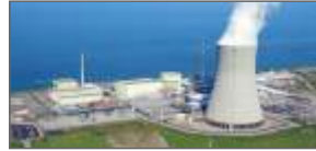
Nuclear Power Stations
