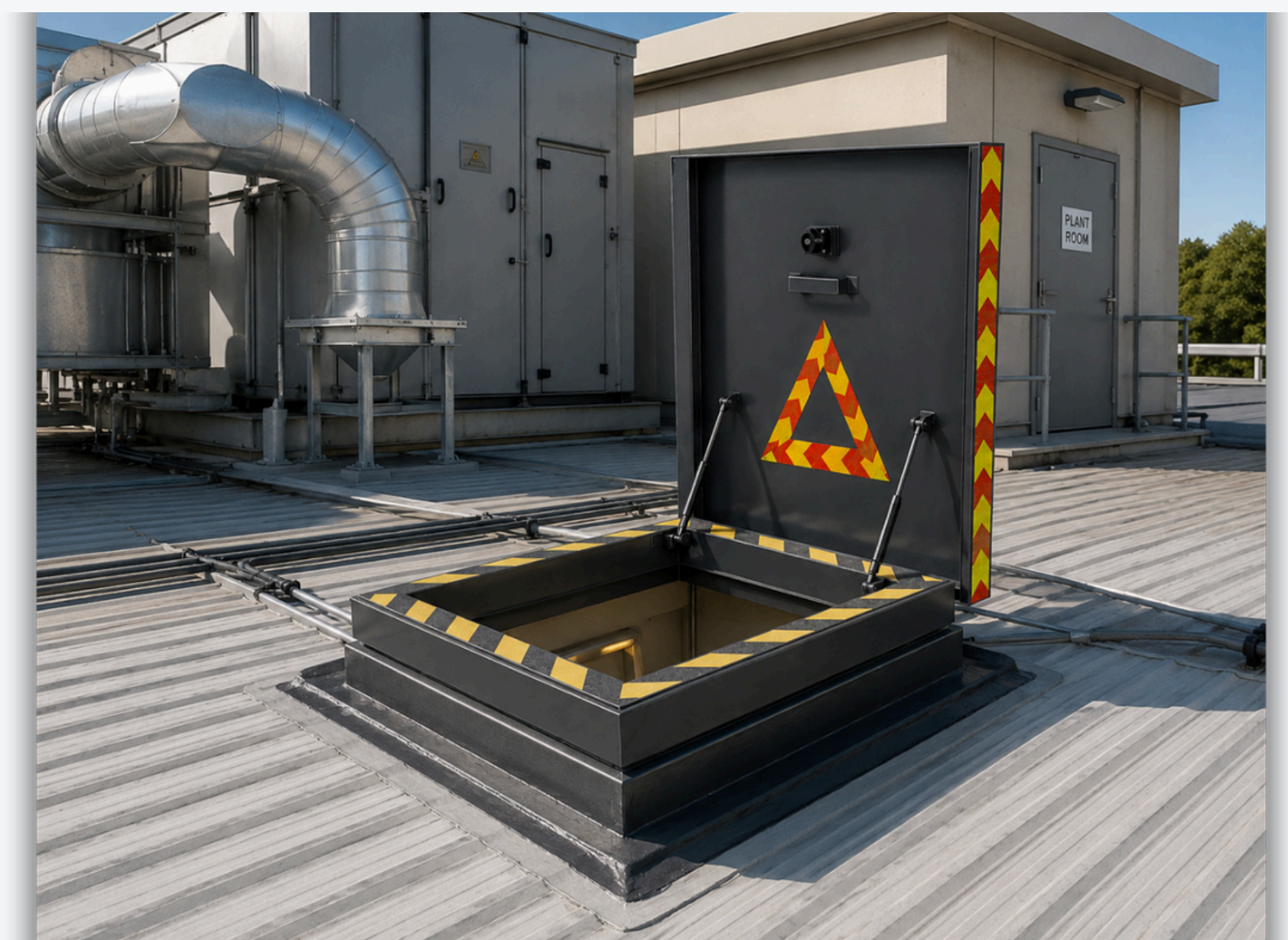
Roof access hatch — plant-room roof, installed
