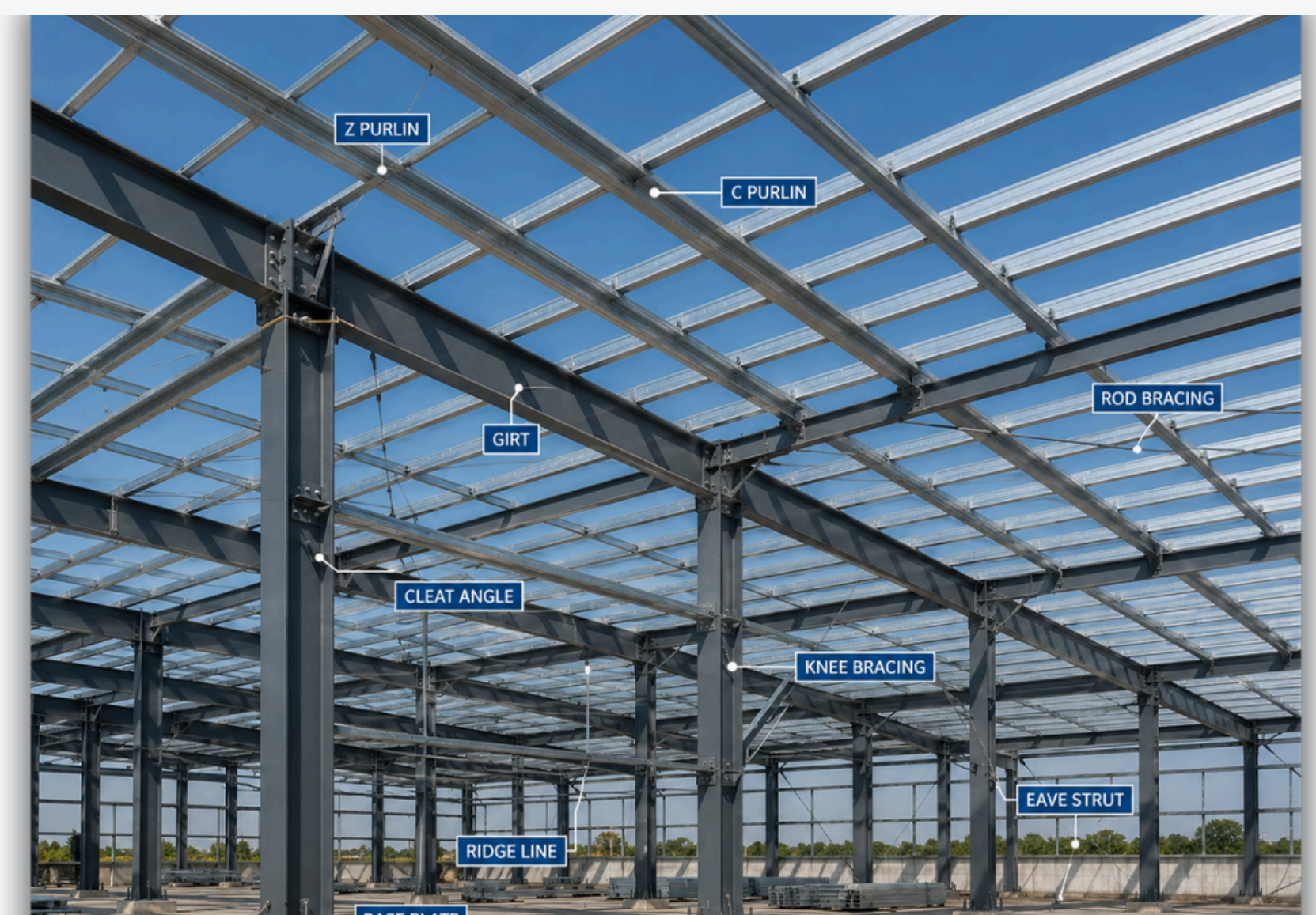
Purlins & structural accessories — support framework
