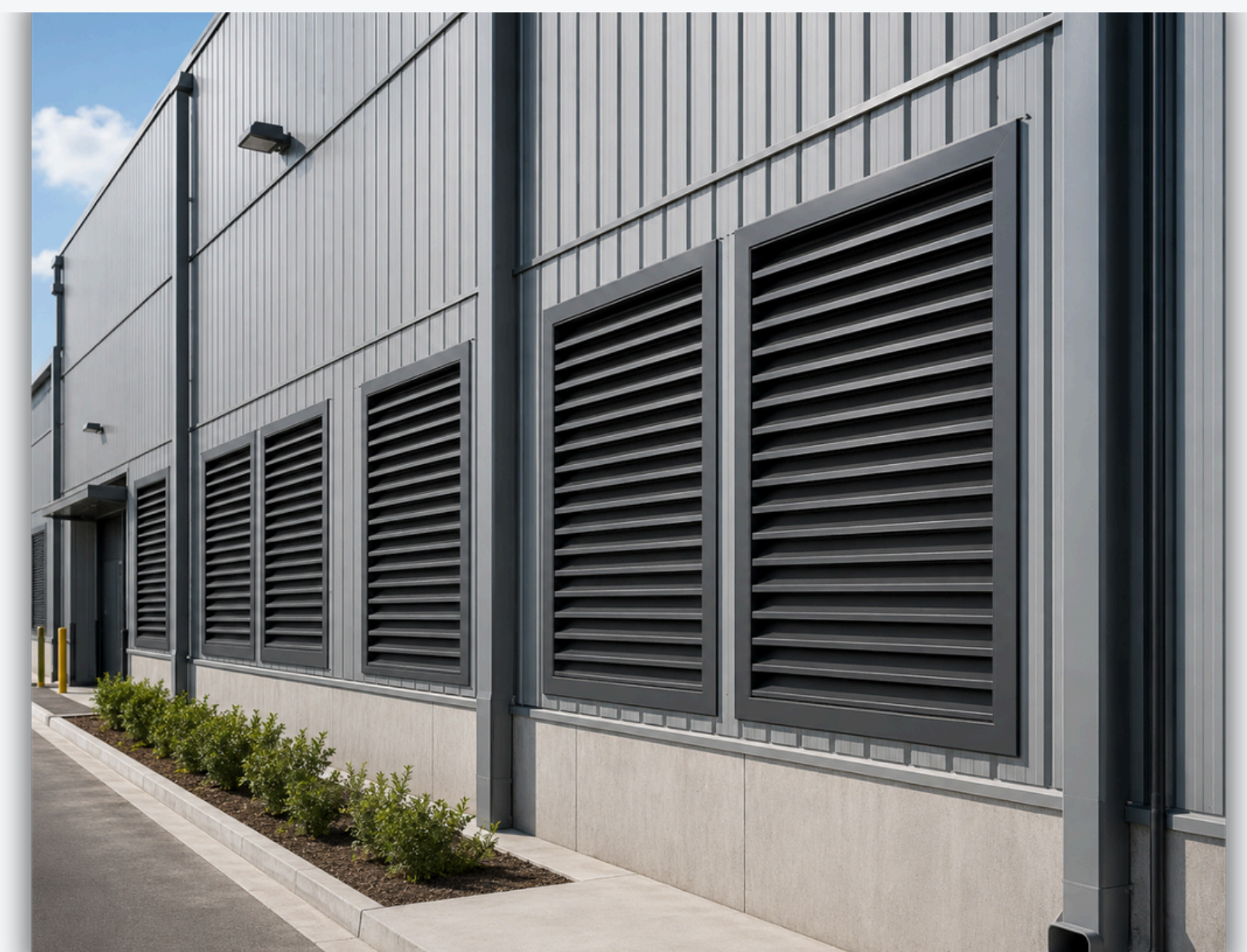
Aluminium louvers — industrial facade installation
