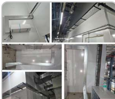
HVAC Cable Tray
