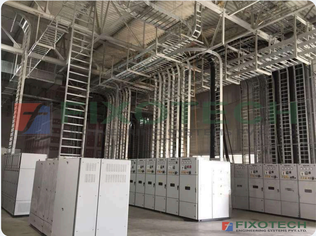
MULTI-TIER LADDER & PERFORATED TRAY RUN — INDUSTRIAL FACILITY CEILING GRID
