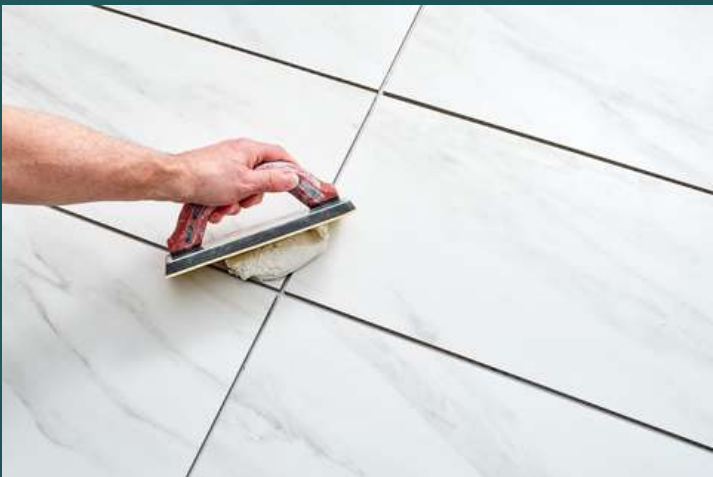
Sealer Grout Applying on Tile
