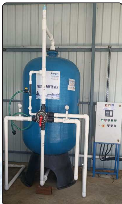
MSEP Rubber Lining Water Softening Plant
