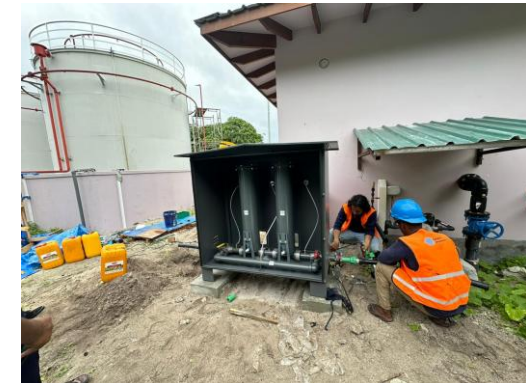
Filtration System Installation In Fueling Station
