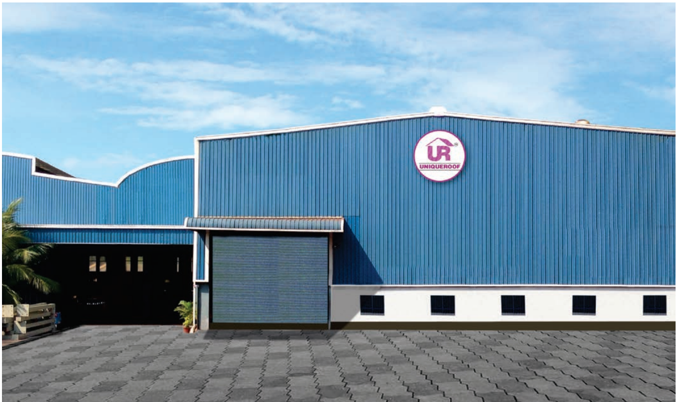
Uniqueroof (P) Ltd - Factory - Coimbatore
