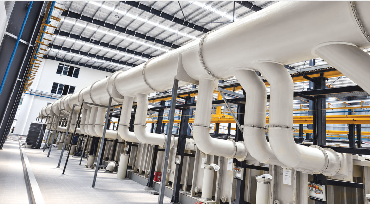
PP+FRP Ducting is designed for the safe extraction and transportation of corrosive fumes, chemical vapours, gases, and contaminated air in industrial and laboratory applications.
