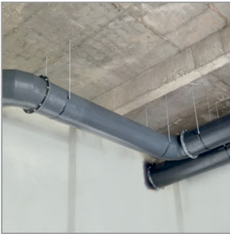
PP+FRP Ducting is designed for the safe extraction and transportation of corrosive fumes, chemical vapours, gases, and contaminated air in industrial and laboratory applications.
