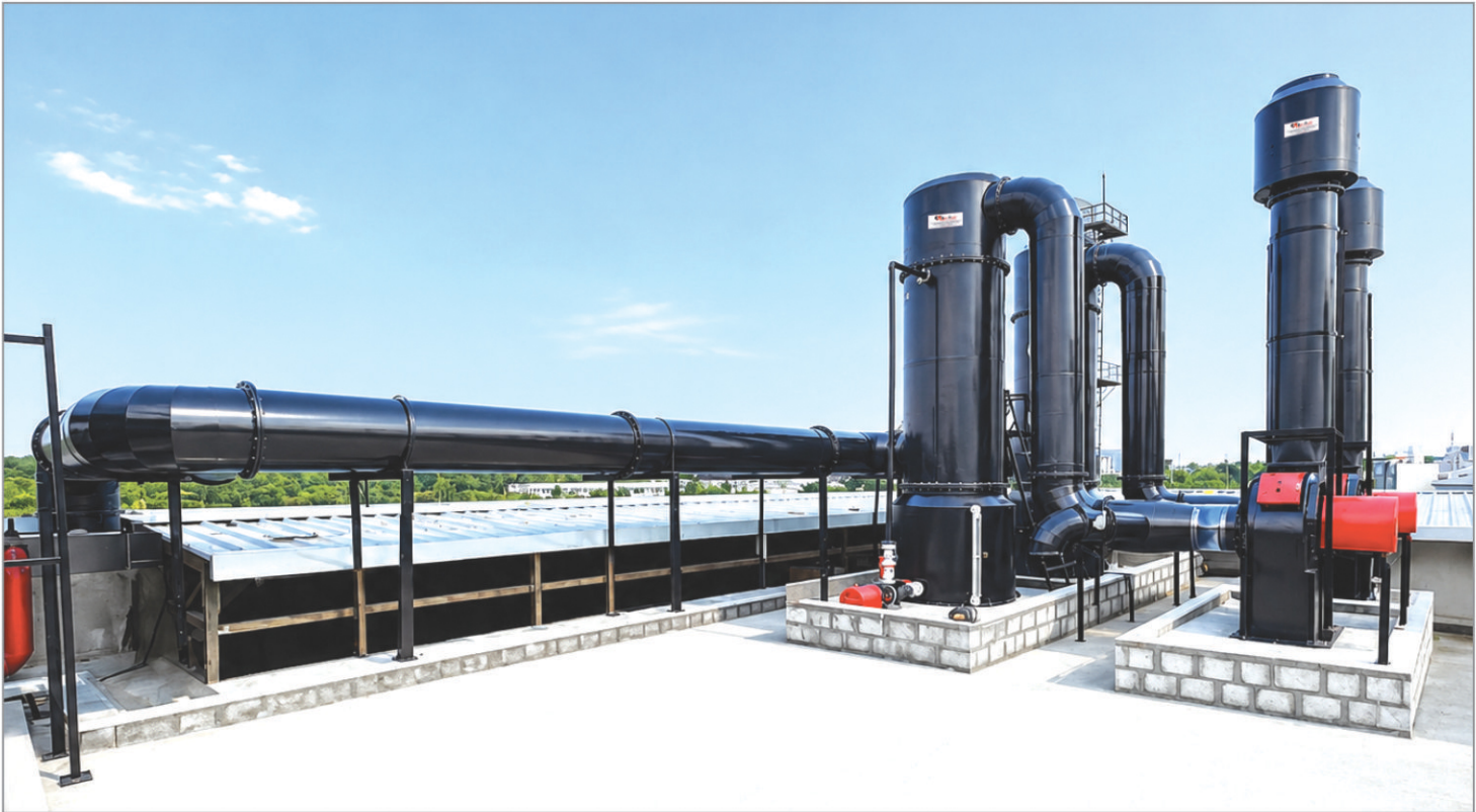
Wet Scrubber System is designed to remove corrosive acid fumes, harmful gases, chemical vapours, odours, and fine mist from industrial exhaust air before discharge into the atmosphere.
