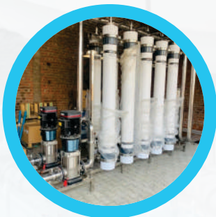
Ultra Filtration 'Plant' ( UF Plant )
