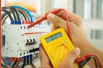
Transformer Testing Services
