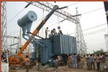
Transformer Erection Commissioning
