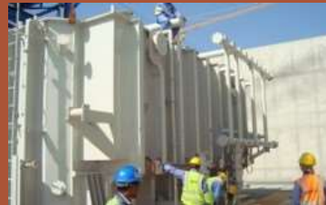
Transformer Commissioning and Testing
