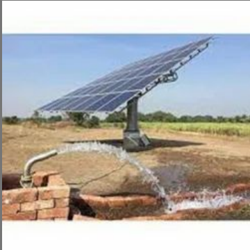
Solar Irrigation System
