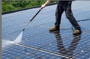
Solar Power Plant Maintenance
