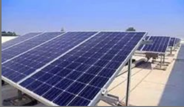
Solar Panel Installation
