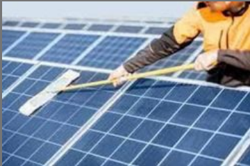
Solar Panel Maintenance Service
