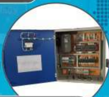
PLC-HMI PANEL
