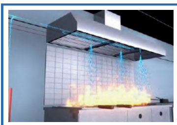
Kitchen Fire Suppression/Flooding System
