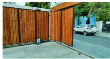
Sliding folding gates are a space-saving gate solution that combines the sliding and folding mechanisms. These gates slide along a track and then fold up to open or close, making them suitable for areas with limited space.
