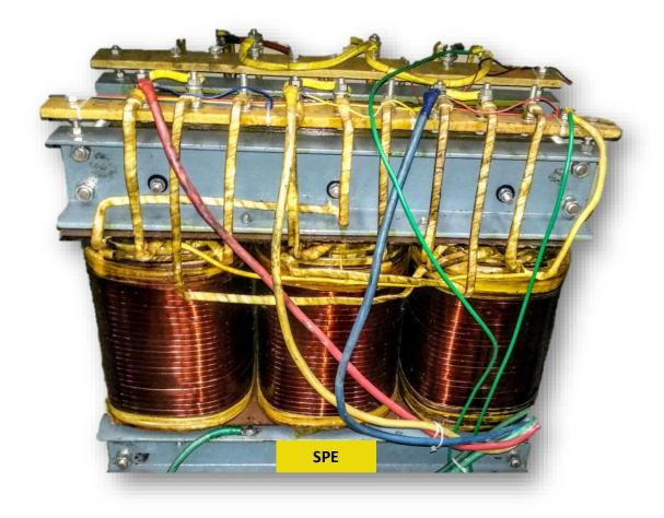
100KVA, 3Ø K-rated transformer I/P: 415V, O/P: 415V
