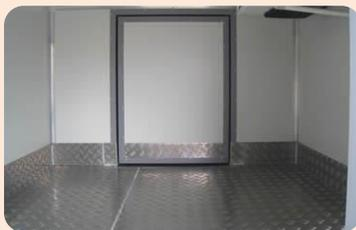
Useful to provide the result of an insulated regular floor and also to form a stable base for wall and partitions.
