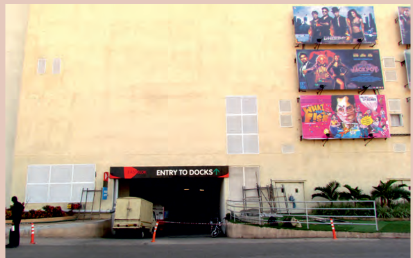
Weather Louvers - Installation at Site
