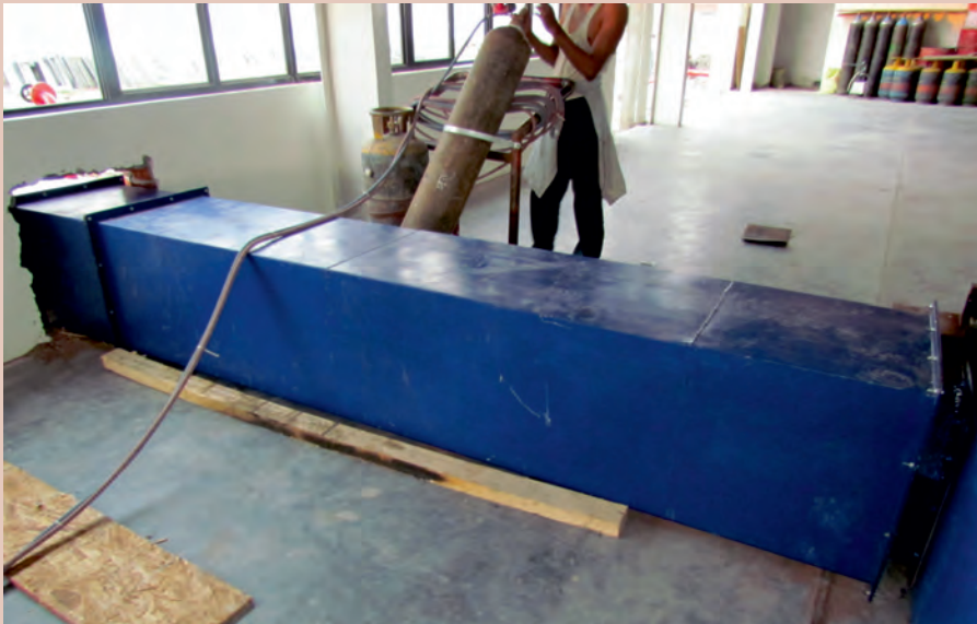
M.S. Ducting & Installation at Site
