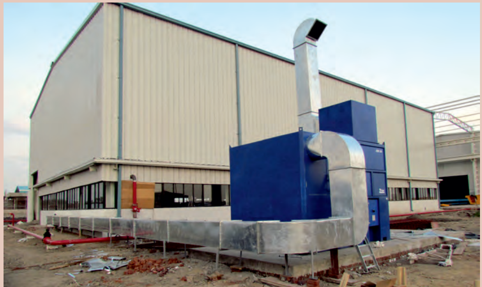
G.I. Ducting & Installation at Site
