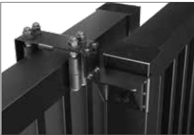
Panel guide to hold both panels when gliding for safety (for double panel type)
