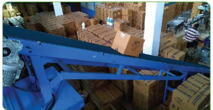
Inclined Belt Conveyor
