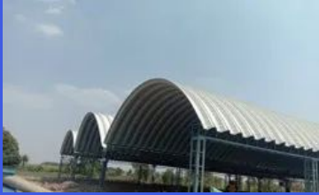
Stainless Steel Roofing Structure
