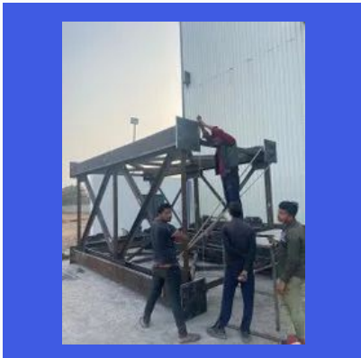
Heavy Industrial Fabricator Service
