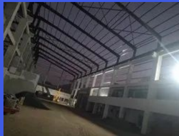
Industrial Peb Structure Erection Work
