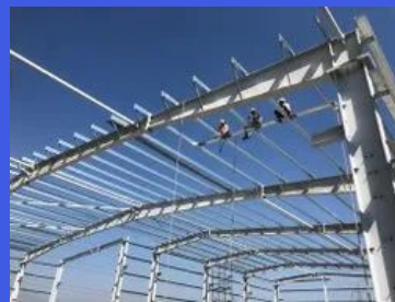
Roofing sheet Shed
