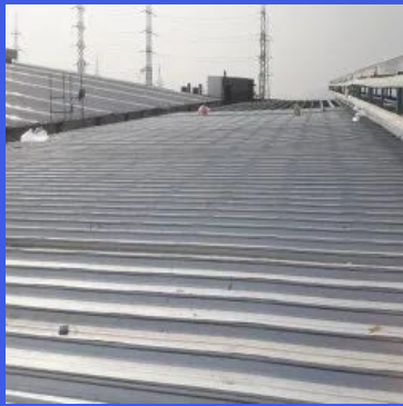
Standing Seam Roofing
