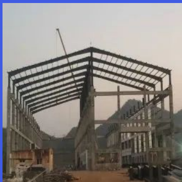
Steel Prefabricated Industrial Structure
