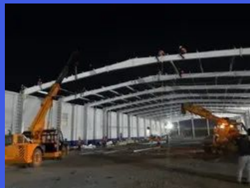
MS Industrial Shed Structure
