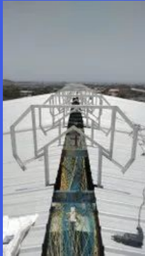
Roofing Sheets Instalation Services
