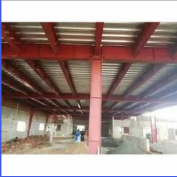
Decking Roofing Sheets Installation Service
