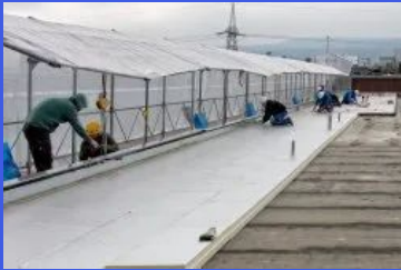
Thermal Insulation Roofing Sheets Installation Service
