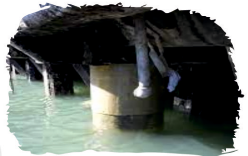
under water chemical treatment
