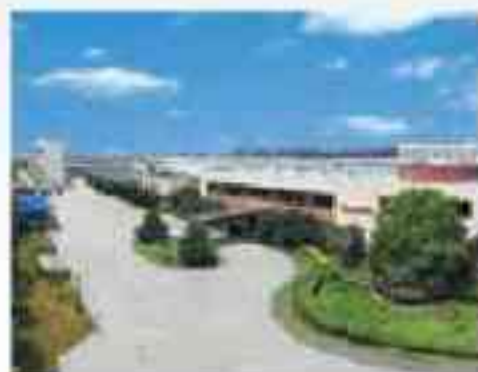
China Plant (MCC)
