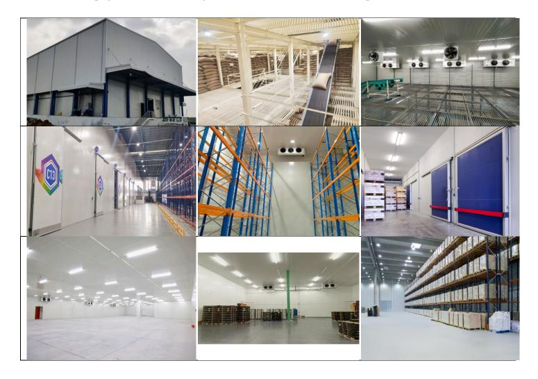
**Puf Panels,** also known as Polyurethane Foam (PUF) panels, are commonly used in cold chain applications due to their excellent thermal insulation properties. Here some of applications of Puf panels in the cold chain industry:
