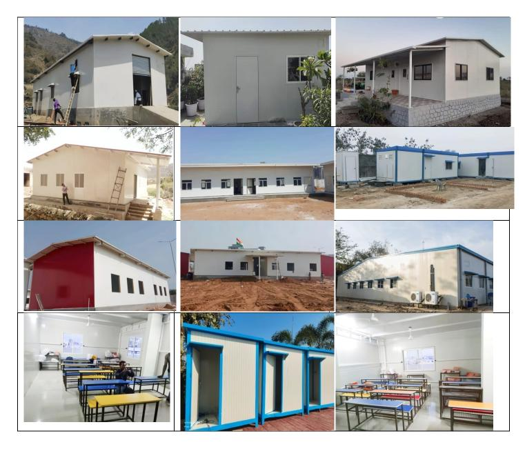
Prefabricated shelters are pre-built structures designed to provide protection, cover, or accommodation in various environment. These shelters are constructed off-side in factory and then transported to their intended locations for assembly. Prefabricated shelters are versatile and can serve a wide range of purposes some of them are:-
