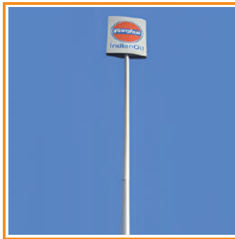
Petrol Pump Pole
