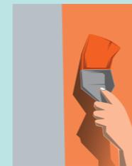
Apply 2-3 coats of Asian Paints Ace/Apex by diluting 1 litre with a maximum of 400 ml of water. Ensure a gap of 4-6 hrs between the coats. Apply a third coat on horizontal surfaces for additional protection.
