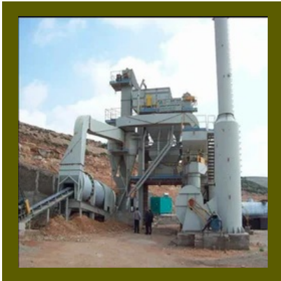
Asphalt Hot Mix Batch Plant
