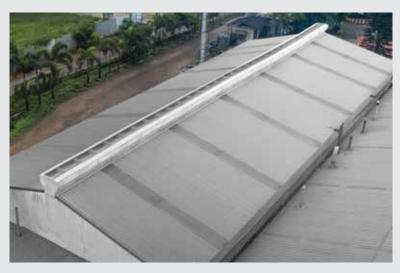
Protected monitors (side openings are protected against wind) where the final exhaust opening is top facing and the air path through the ventilator is precisely defined for minimum friction losses. made by Gravent.
